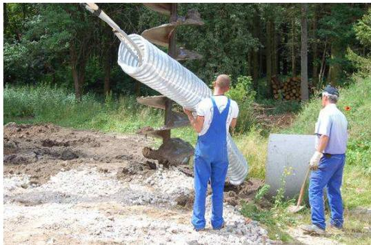
Fig. 3: Inserting the probe
