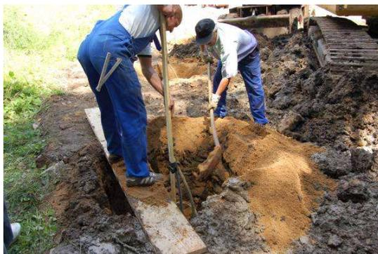
Fig. 4: Filling the borehole
